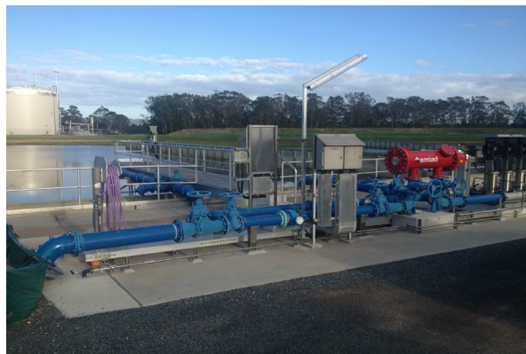
Wastewater Treatment Plant, Coombabah
